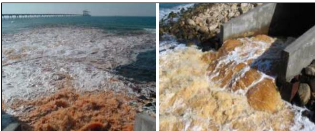
Figure (C.1): Ashkelon`s onshore open channel disposal system
